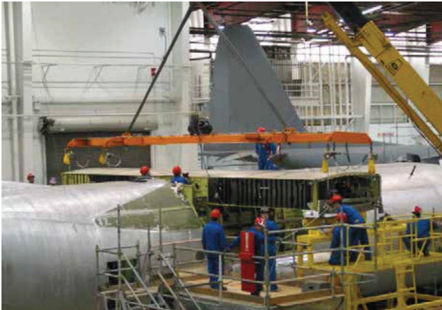
Figure A-3 Positioning a C-130 Centre Wing
