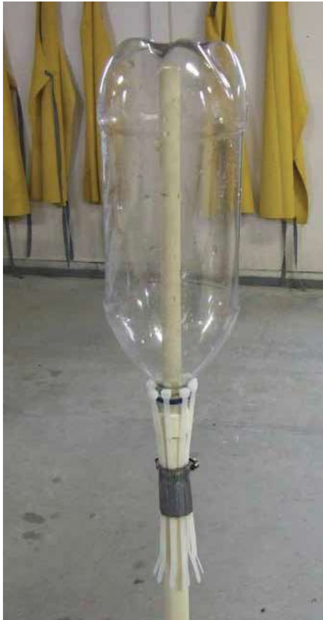
Figure 24-A Cable Ties Holding the Soda Bottle
